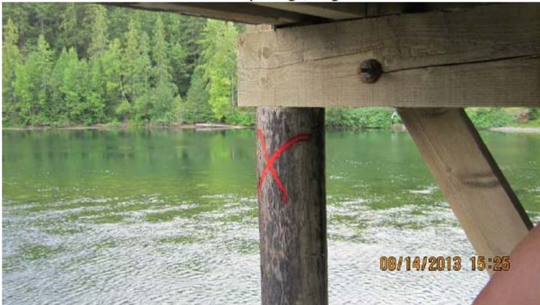
Photo 14. Likely Bridge, August 2013
